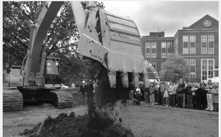
Purdue President Martin C. Jischke uses a Caterpillar back-hoe to break ground for the Neil Armstrong Hall of Engineering at a ceremony Oct. 16. (Purdue News Service photo/David Umberger)
